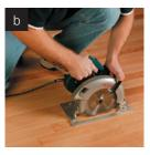
Using a circular saw or router, cut the board lengthwise to within 1/2" of the edges. For a glued board, make several cuts close together to separate the board into smaller sections.
