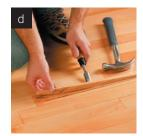
Using a wood chisel, remove the central part of the board first (between the side cuts).
