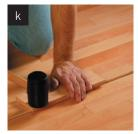
Install the board, using a rubber mallet and a wood block to place it in position.
