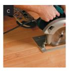
Make a diagonal cut down the center of the board from one end to the other of the cuts made in Step B. It may be necessary to make more than one cut if the board is glued in place.
