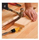
Remove nails or staples (this step does not apply to glued Engineered boards), then remove edges, taking care not to damage the adjacent boards.
