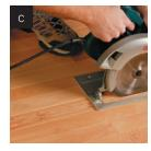
Make a diagonal cut down the center of the board from one end to the other of the cuts made in Step B. It may be necessary to make more than one cut if the board is glued in place.
