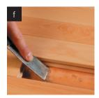
Remove the underlying construction paper or adhesive and clean any residue from the subfloor.
